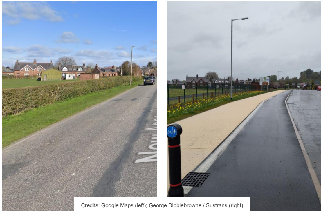
Figure 8: Grass verge before (left) and new segregated cycle/foot path after (right) the infrastructure changes
