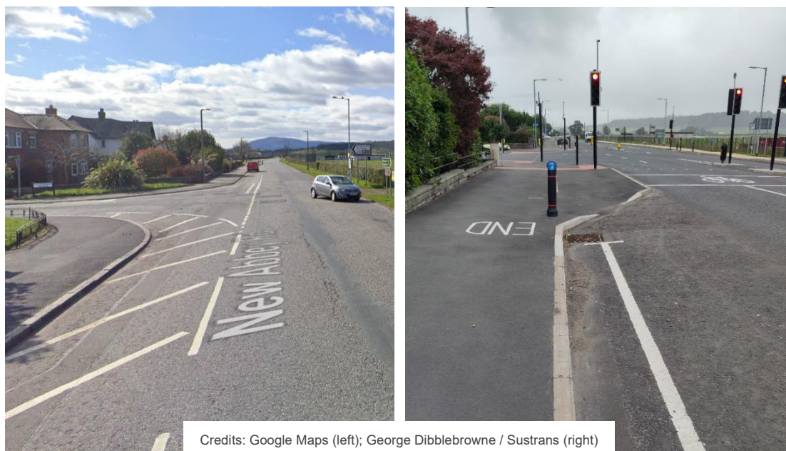
Figure 6: Pleasance Avenue junction before (left) and after (right) the infrastructure changes
