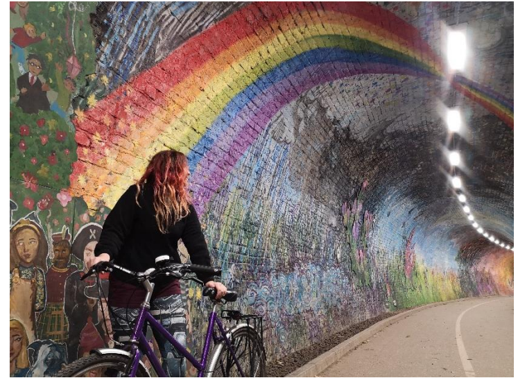
A dark and scary tunnel transformed, 2020
