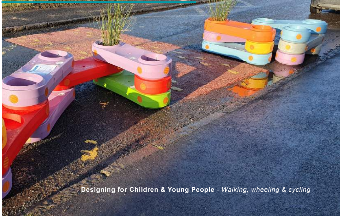
Temporary build-outs installed for trials (street kit)
