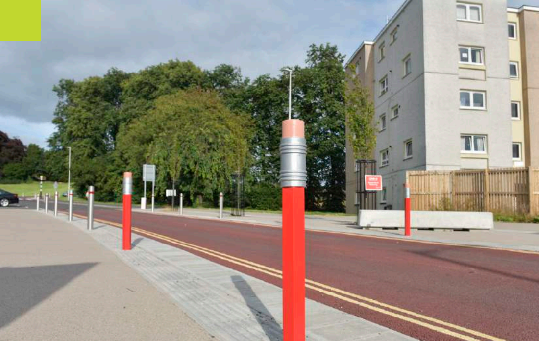
Red asphalt and playful bollard preventing pavement parking
