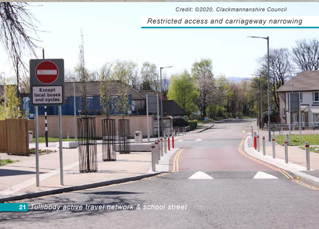
Red asphalt and playful bollard preventing pavement parking
