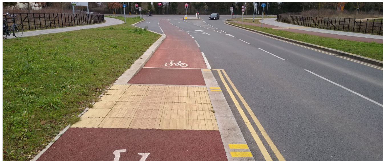
Figure 23. Transition from cycle track (footway level) ramped to cycle lane (carriageway level)
