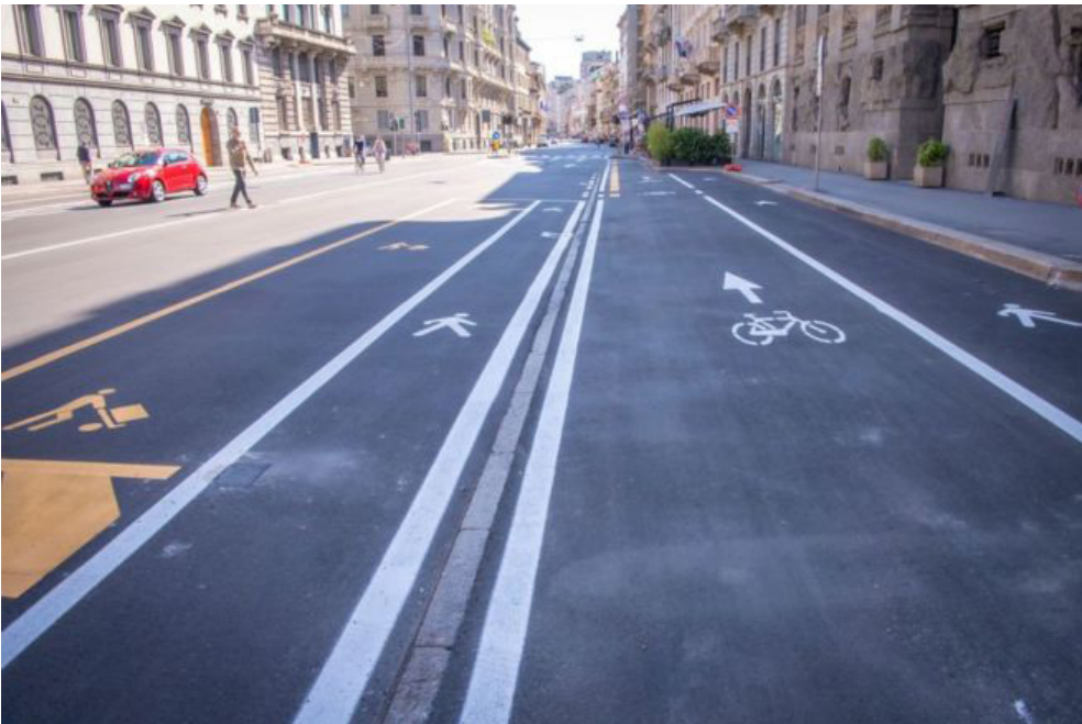
Figure 30. Example of layout to accommodate loading alongside cycle lane in Milan
