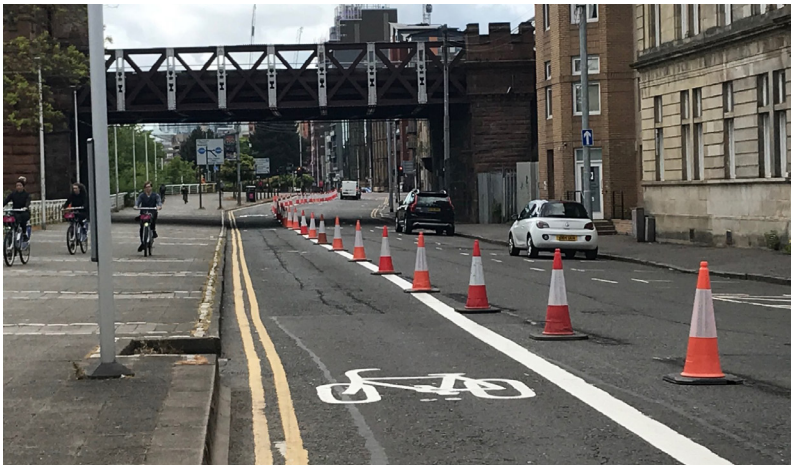
Figure 4. Carriageway converted into temporary cycle lane, Glasgow
