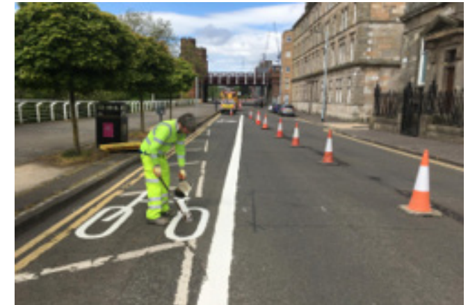
Figure 39. Marking out new cycle lane
