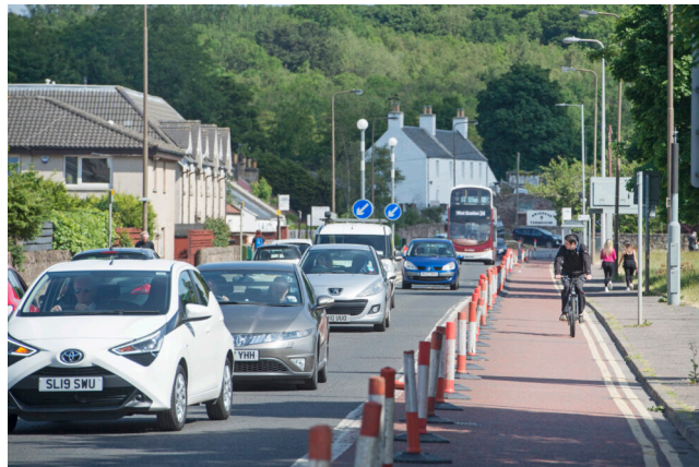
Figure 1. Lane separators along Old Dalkeith Road in Edinburgh. These ensure the cycle lane remains free of parked vehicles for key workers whilst still allowing access to resident driveways.
